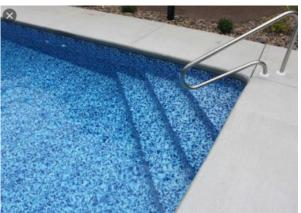
Note: The permanent cement step width about 3.5 meters and deep 1.5 meters including around 4-5 steps
